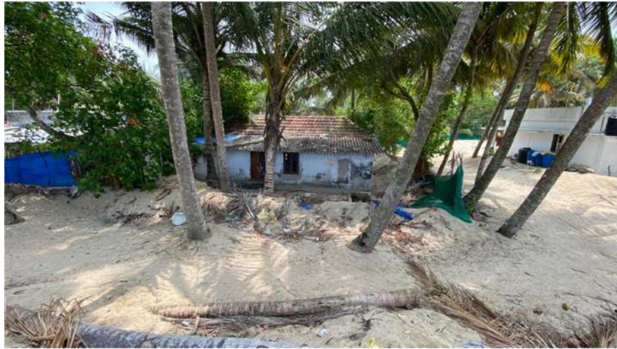
Fig.1. Sand deposits inside residential area which leads house uninhabitable
