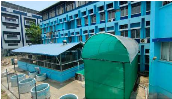
Fig 1a. Hatchery facility
