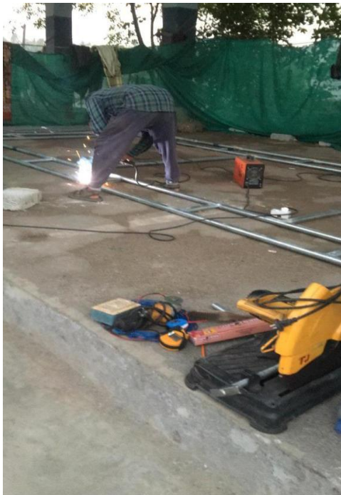
Construction of fish cages at Anappuzha
