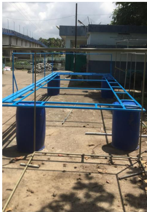
Construction of fish cages at Anappuzha
